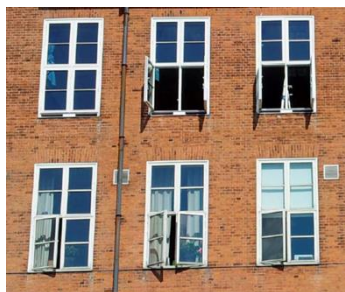
New windows with integrated air inlet and outlet in the frame
