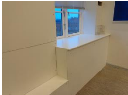
Grøndalsvænge School in Copenhagen. Window integrated heat recovery ventilation from Ecovent.
